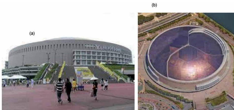
Figure 1. (a) Aerial approach view of the Fukuoka dome, built in 1993, which is covered with (b) titanium roofing, retractable for multi-role and all-weather purposes.
