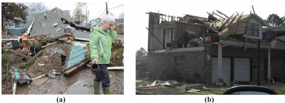
Figure 1. Hurricane-induced damage: (a) complete collapse of a residential home induced by hurricane Sandy, New York, 2012 [8] and (b) severe roof damage by hurricane Rita in Lake Charles, in 2005 [9].
