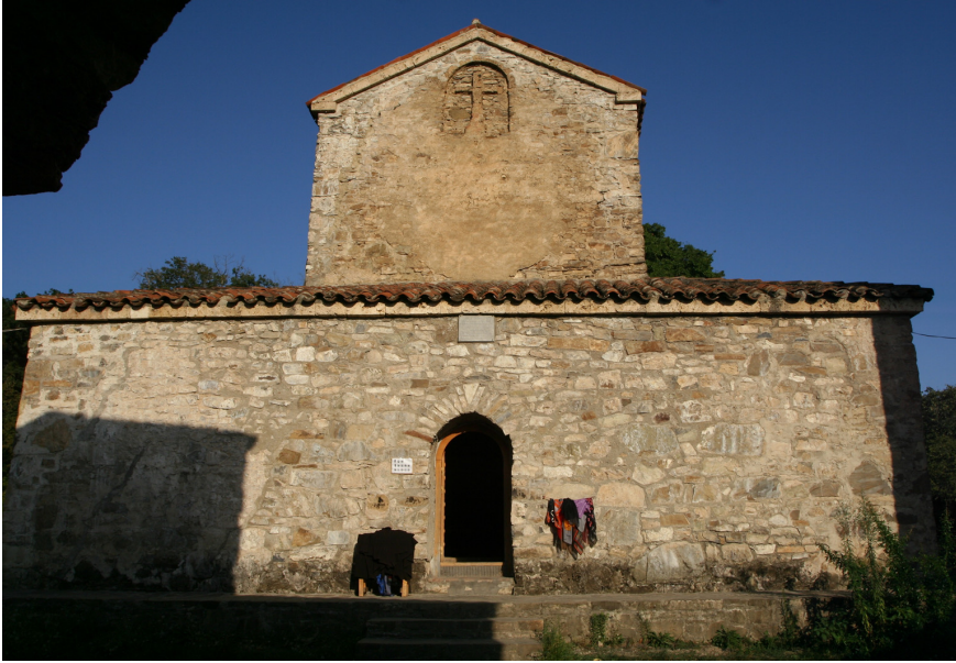
FIGURE 18 West façade of the sixth-seventh century basilica at Nekresi
