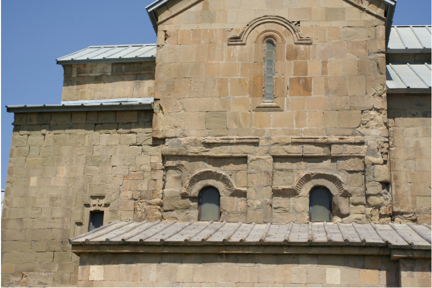
FIGURE 14 South façade of Tsilkani with decorative bands over windows
