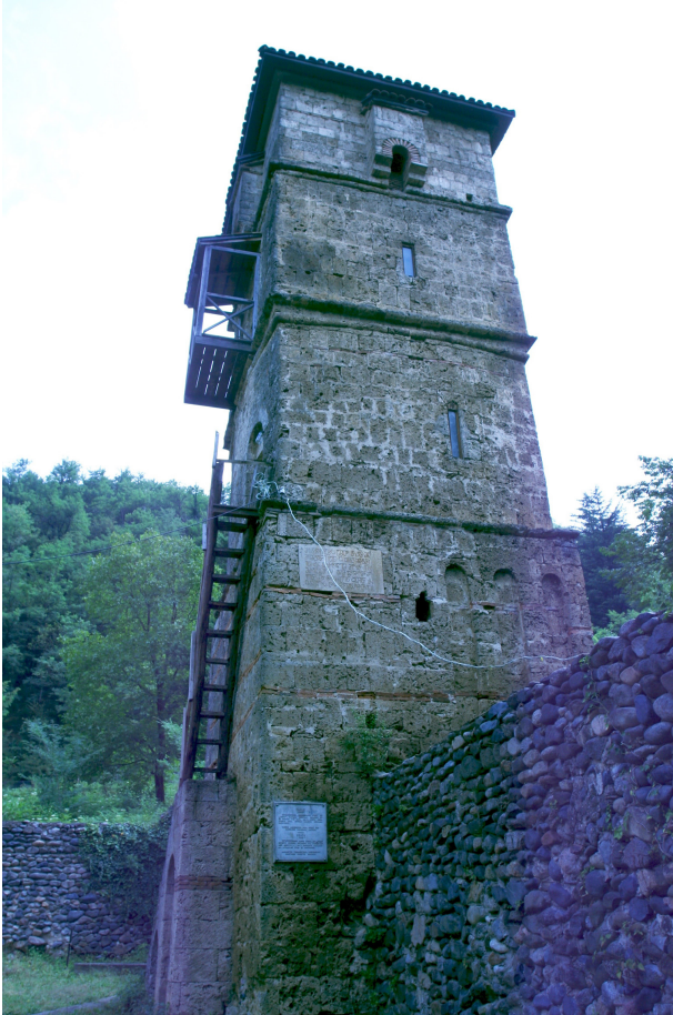
FIGURE 12 'Stylite' tower house at Ubisi
