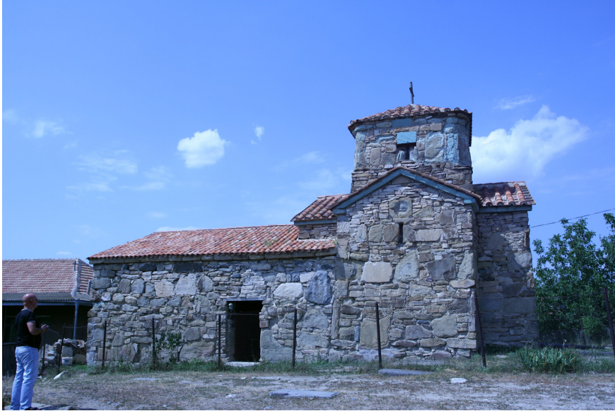
FIGURE 23 Idleti, southern façade showing extended narthex
