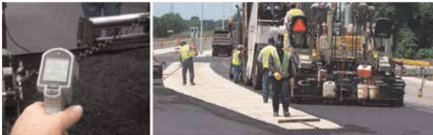
Figure 5. Low temperature of production for warm mix asphalt (courtesy of Federal Highway administration).
