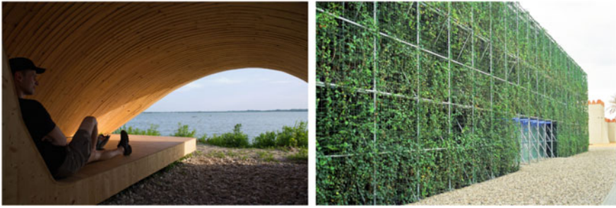
Fig. 7.2 Different approaches for connection with nature. Duna Building (Bergen School of Architecture, Slovak University of Technology in Bratislava), photograph courtesy of Veronika Kotradyová (left) and Romanian Pavilion at the World Expo 2000, arch. Doru O. Comsa, 2000 (right)
