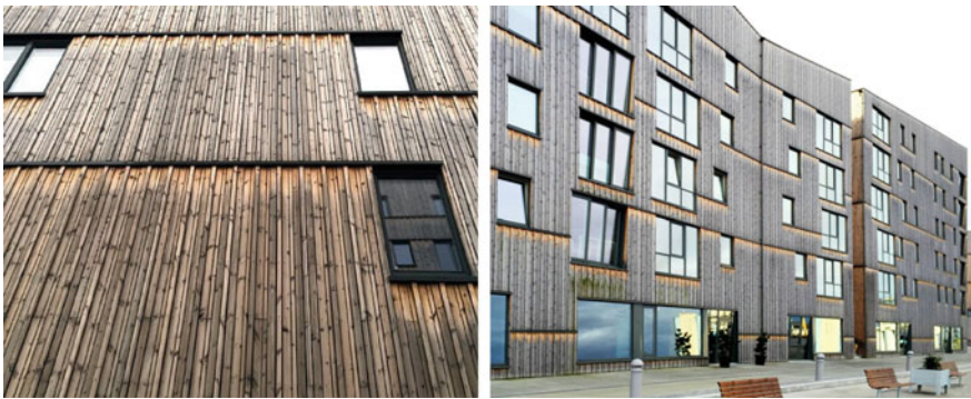
Fig. 5.3 Weathered building in Stavanger, Norway. Image courtesy of Lone Ross Gobakken, NIBIO
