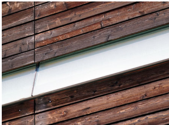
Fig. 5.12 Protection by design details allowing fast water run-off. Image courtesy of Lone Ross Gobakken, NIBIO
