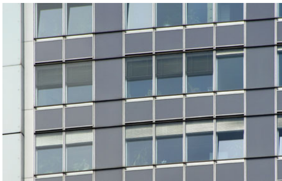
Fig. 1.5 Commerzbank in Frankfurt am main (arch. Foster and Partners, 1997)
