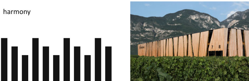
Fig. 3.7 Harmony in architecture and its implementation—the Rotho Blaas SRL company, Cortaccia (BZ), Italy. Photograph courtesy of Rotho Blaas SRL
