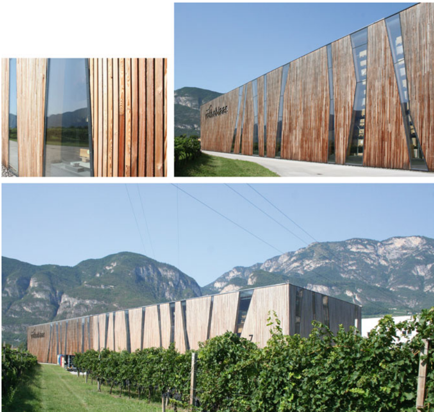
Fig. 4.16 Rotho Blaas SRL headquarters. Photograph courtesy of Paolo Grossi
