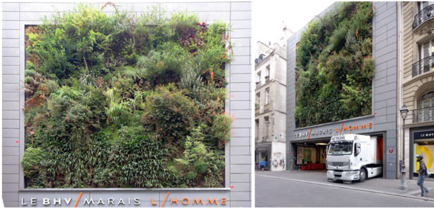
Fig. 2.17 Green wall implemented as a building façade
