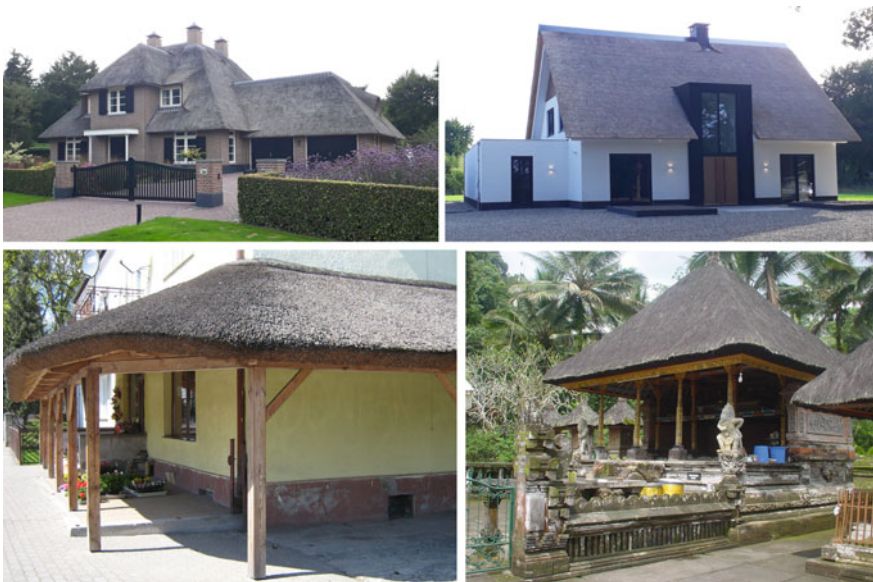
Fig. 2.4 Use of straw in roof coverage
