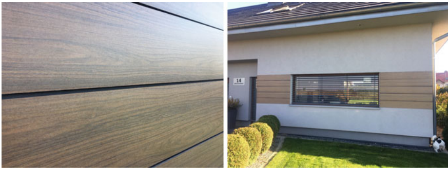
Fig. 2.14 Use of HPL as a building façade. Photograph courtesy of Ewa Osiewicz
