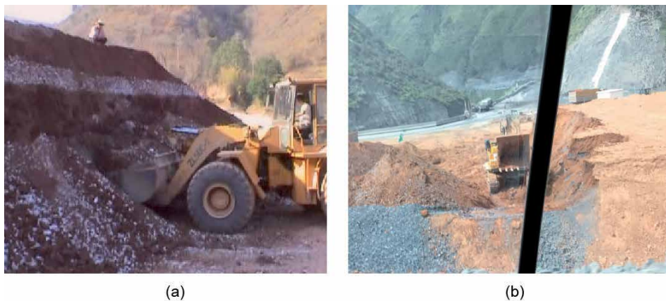
Figure 15. Blending techniques used in the NZD and LHK dams. (a) The NZD dam and (b) the LHK dam.
