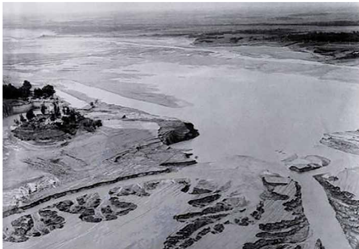
Figure 2. Final breach of Shimantan dam.
