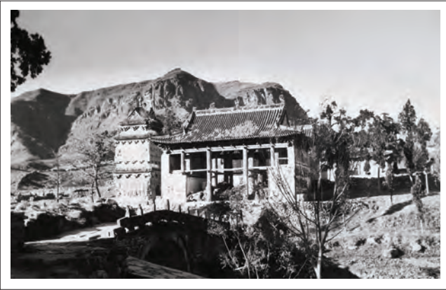
Figure 31.7 Temple of Bian Que, Shentou village 神頭村, Neiqiu 內丘 county, Hebei province. © Ma Kanwen
