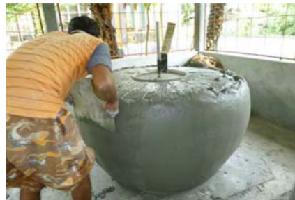
Figure 7.6 Mortar treatment on the mud layer. (Source: Author's own).
