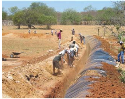
Figure 16.7 Sub-surface dam construction, placing the PVC sheet. (Source: Author).
