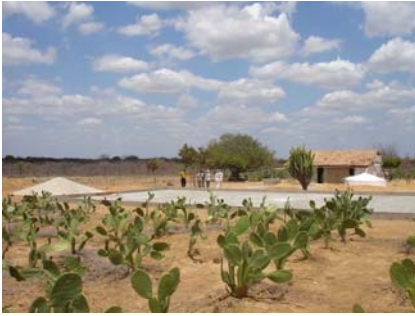
Figure 16.6 Cistern of 52,000 L with catchment area for irrigation of fruit trees and vegetables, near the house a cistern of 16,000 L with drinking water. (Source: Author).
