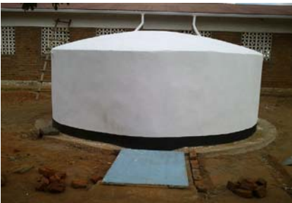
Figure 11.4 30,000 L ferro-cement tank Kasungu District. (Source: Author's own).
