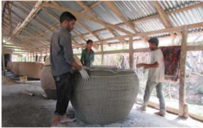
Figure 7.7 Reinforcement with wire net. (Source: Author's own).
