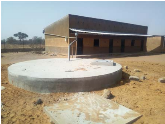
Figure 10.2 Rainwater harvesting system in Dekhaye School. (S.Sene, 2018).
