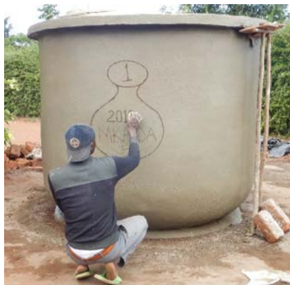
Figure 18.6 Finishing the outside. (Source: Author's own).
