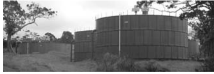
Figure 4.7 A few of the larger potable water storage tanks for Kilauea Military Recreational Camp.
