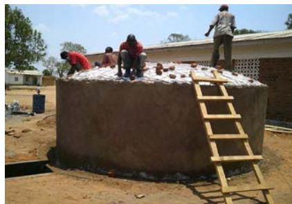
Figure 11.5 Ferro-cement tank under construction. (Source: Author's own).
