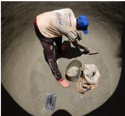
Figure 18.5 Finishing inside a calabash cistern. (Source: Author's own).
