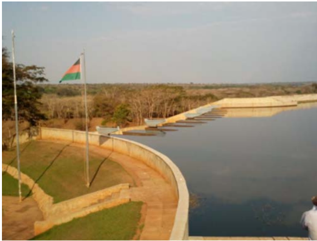
Figure 11.10 Communally owned earth dam, Chitsime EPA, Lilongwe district. (Source: AMEI (2014)).
