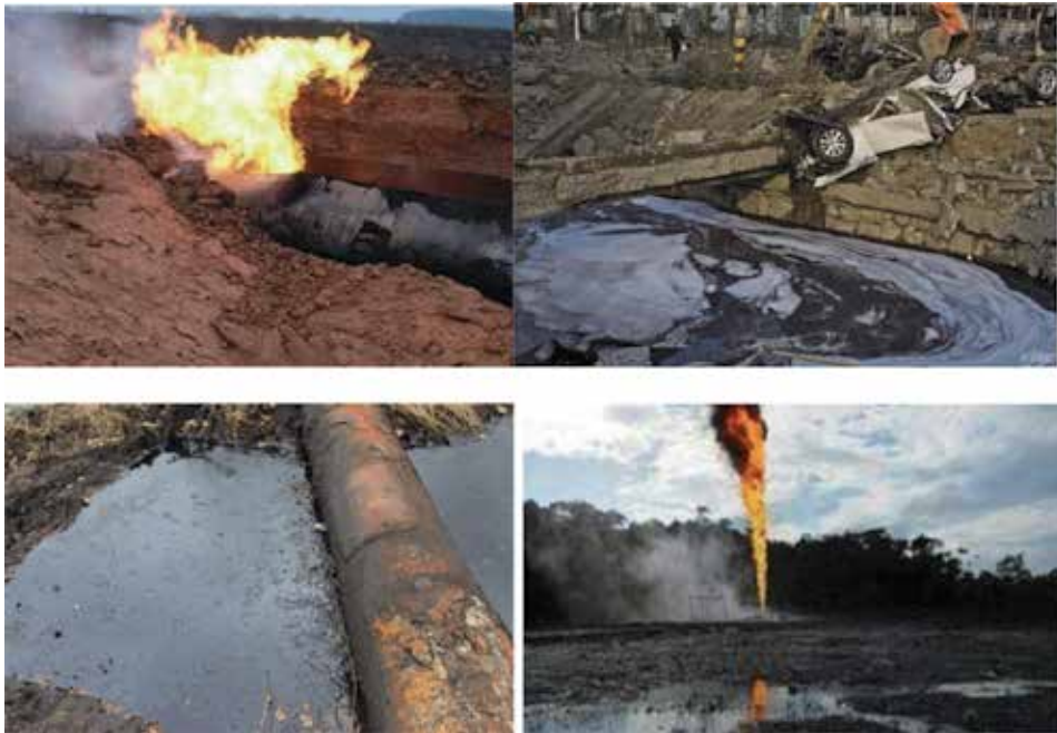
Figure 2. Accidents on oil pipelines (Venezuela, China, Russia).
