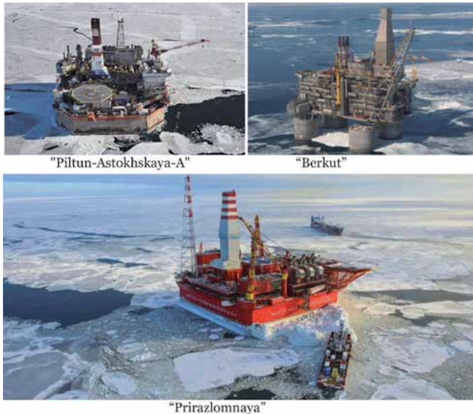
Figure 1. Large offshore platforms in Russia.
