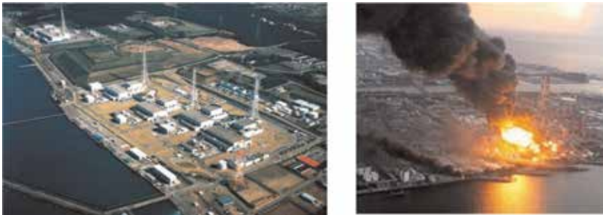
Figure 4. The accident on the “Fukushima-1” NPP.
