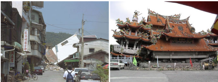
Fig. 12.5 Collapsed buildings (L) and Wuchang temple (R) in Chi-Chi, Taiwan, due to the 1999 Chi-Chi Earthquake (Murao 1999)
