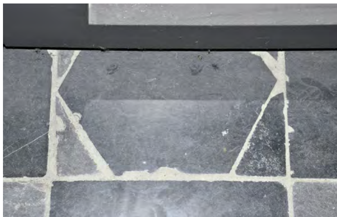
FIGURE 40 Hexagonal cut-away in the floortiles of Saint Leonard's chapel, Zoutleeuw, church of Saint Leonard
