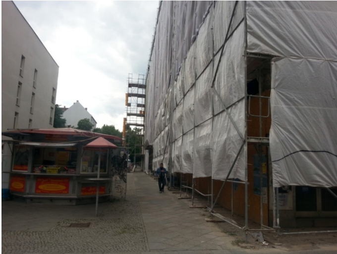
Fig. 32 Building under construction
