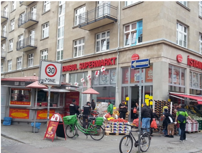
Fig. 33 Upgraded building with new supermarket
