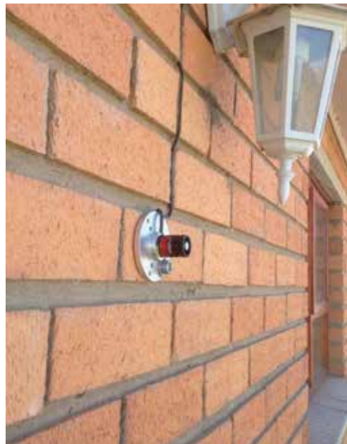
Figure 5. Li-Cor 200R pyranometer for monitoring global vertical irradiance on the east elevation of the passive solar house.
