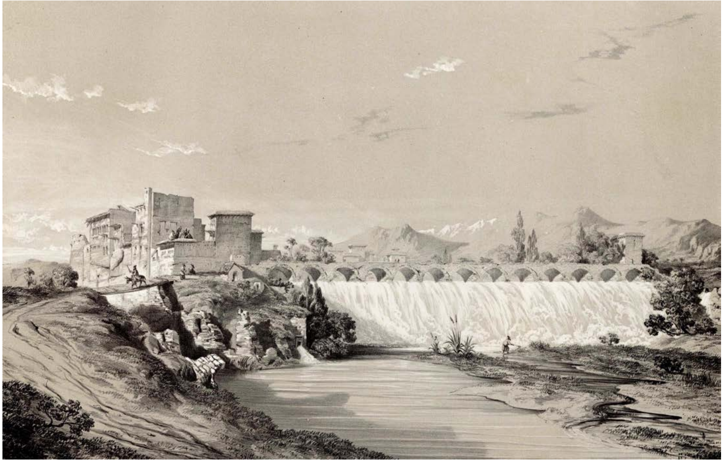
Figure 56: Bridge over the Bendemeer Stream by Coste.
