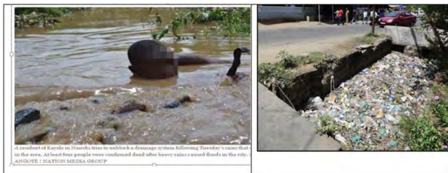
Fig. 4 Poor solid waste management has aggravated inundation in Nairobi
