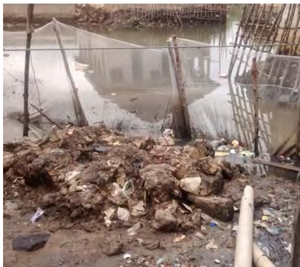
Fig. 9 Nets installed in Baptist waterfront community to protect from waste flowing back into the community (photo credit CMAP 2017)
