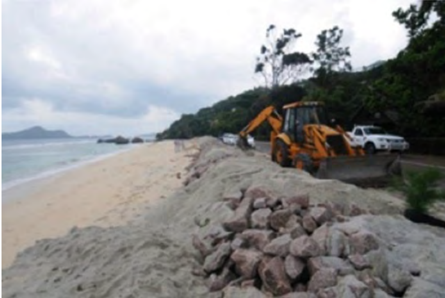
Fig. 6 Beach nourishment project at the North East Point beach, Mahé Island (MEECC 2019)
