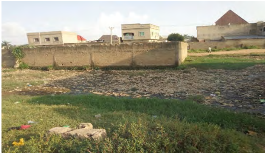
Fig. 6 Abandoned development in a low-lying area due to adverse effect of flooding in the study area (Kofar Ruwa quarters). (Source: Field Survey 2019)
