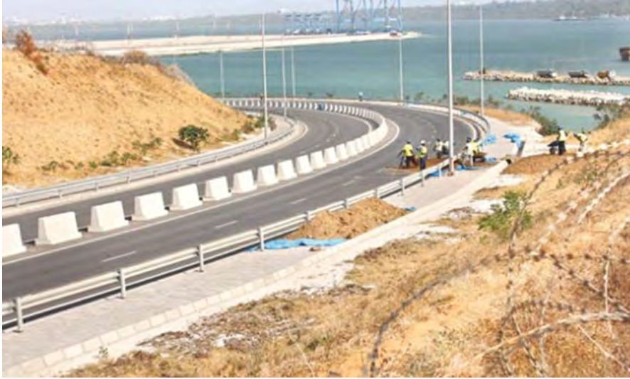
Fig. 5 The new Mombasa road by the seaside in Mombasa city
