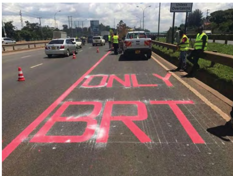
Fig. 7 Lanes marked on Thika superhighway for BRT buses to be introduced by the Kenyan Government in early 2019
