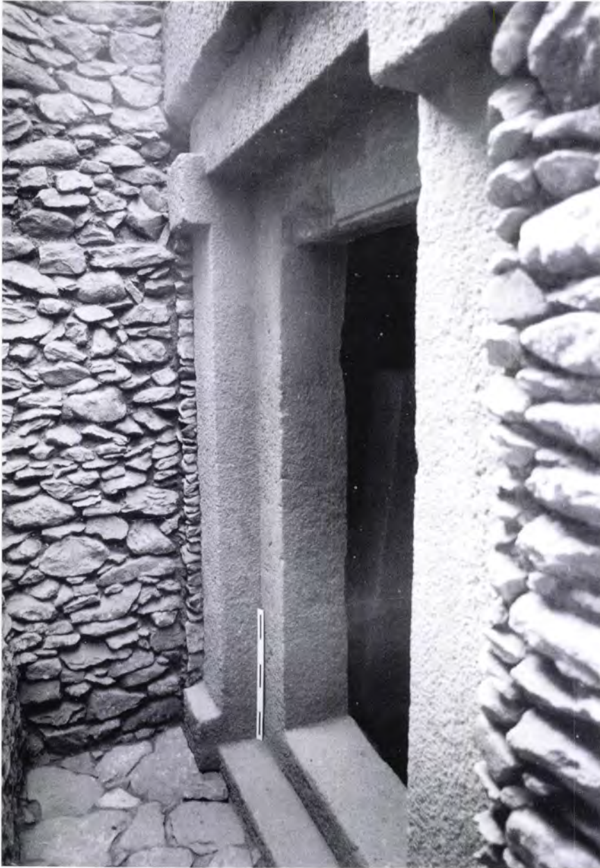
Fig. 137 The eastern portal of the Mausoleum. Scale: 0.5 m.
