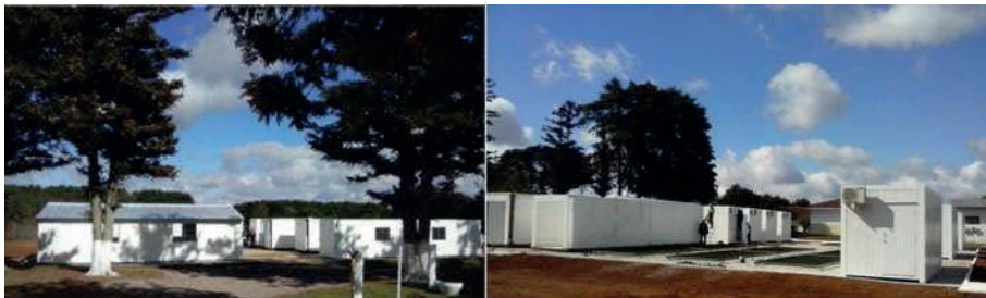
Figure 4. Containerized rearing modules installed for the establishment of the Moscasul Biological Control and Integrated Fruit Fly Management Center at Vacaria, Rio Grande do Sul, Brazil.
