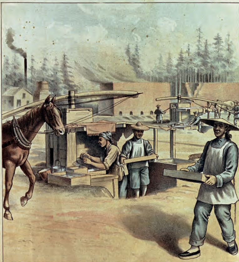
BRICK MAKING, NEAR PORTLAND, OREGON.
