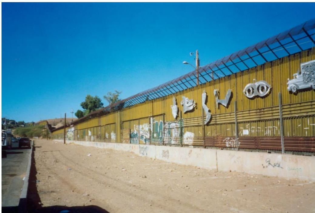
Nogales, Mexico. The infamous steel fence (photo by Millicent I. Lim)
