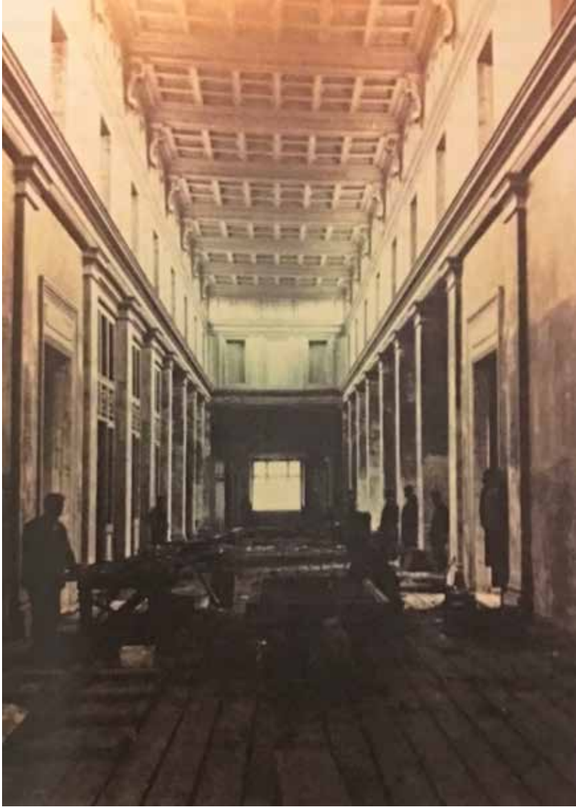
Figure 34 Construction of the new building of the Imperial Museum (1891)
