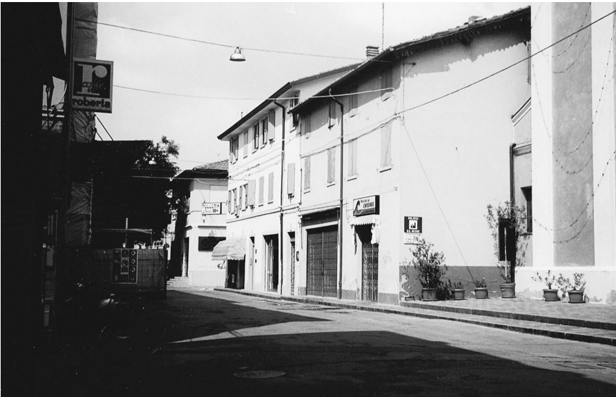
Plate 5 The front left side view of the church
