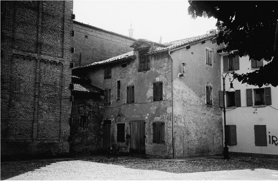
Plate 4 The back left side view of the church
