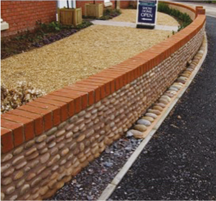
Figure 13.5c Gilbrook estate, Woodbury: new pebble boundary wall (Source: author)
