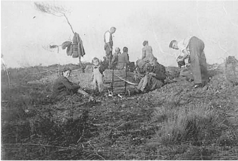
Figure 2.5 Carter's excavation team at work (early 1930s) (Source: Carter archive)
