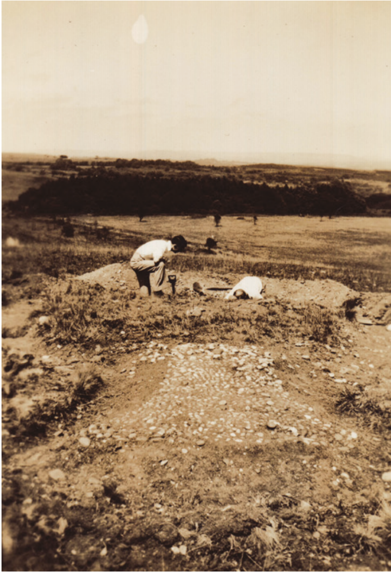
Figure 6.15 Aylesbeare platform no. 1 during excavation, 1937 (Source: Carter archive)
