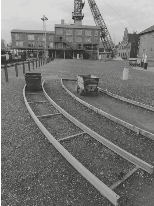
Fig. 9: Aesthetic value of Zollern Colliery architectural monument (author of the photograph I. Tandzegolskienė)
