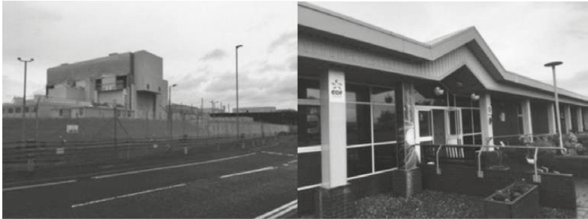
Fig. 2: Torness Nuclear Power Plant and Visitor Center (Photographs by E.Gerulaitienė)
