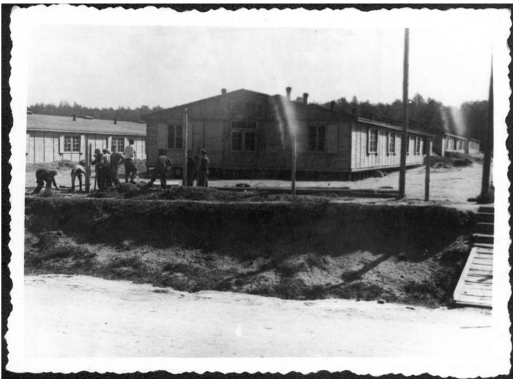
People constructing a barbed wire fence at a labor camp, Poniatowa. Archival signature: 76F06. Yad Vashem Archives.
