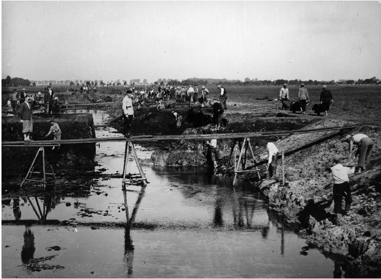
Construction of drainage channels in the Krzna valley in the vicinity of Biała Podlaska. ( Zeitungs-Verlag Krakau-Warschau. ) Archival signature: 2-6918b. National Digital Archives (NAC), Warsaw.
