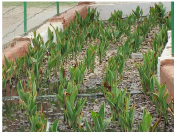
Figure 17.10 Treatment unit planted with Canna indica.
