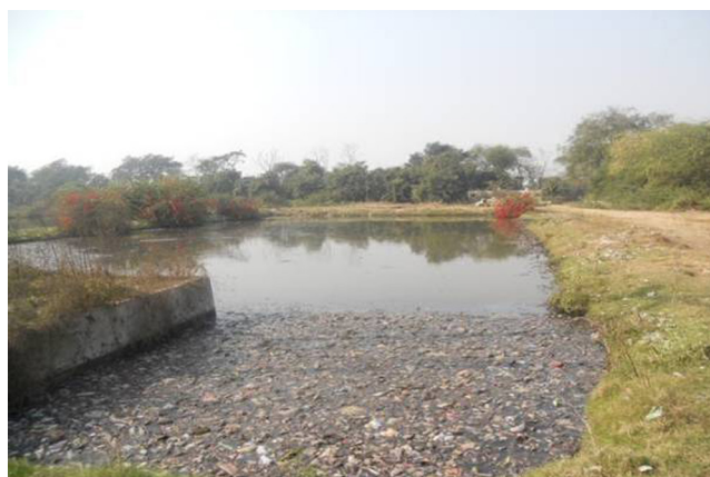
Figure 8.11 Poor maintenance of primary treatment unit lead to carry-forward of garbage and solids in WSP in the Municipal WWTP of the City of Vrindavan.
