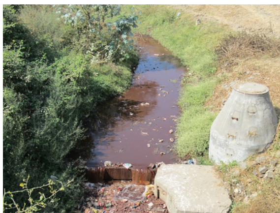
Figure 8.4 Effluent from the textile industry was mixed with domestic wastewater at the inlet of KT-CW in the City of Ujjain, central India.
