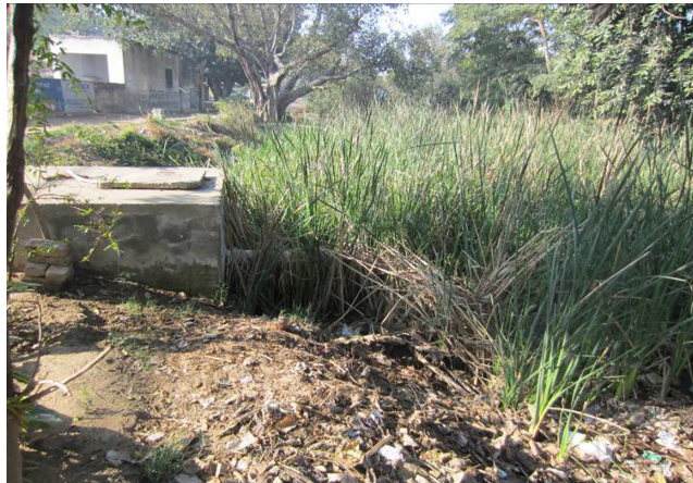
Figure 10.12 Outflow of septic tank connected to the HSSF-CW having Typha latifolia .
