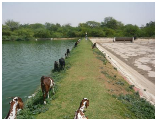
Figure 17.5 Maturation ponds: left side operational, right side not functional.
