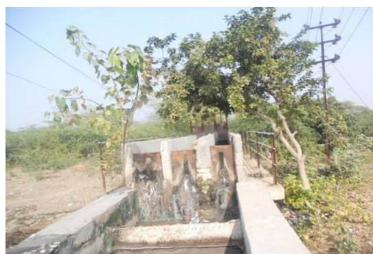
Figure 8.10 Poor maintenance of the primary treatment unit prior to WSP in the Municipal WWTP of the City of Vrindavan, northern India.
