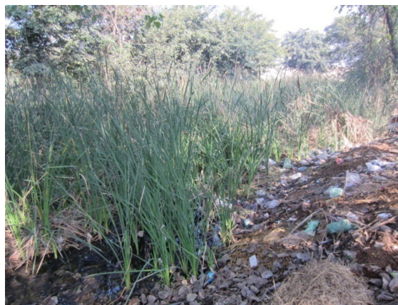
Figure 8.9 Poor maintenance of primary treatment unit lead to carry-forward of garbage and solids in the wetland bed of HSSF-CW in the City of Ropar, northern India.
