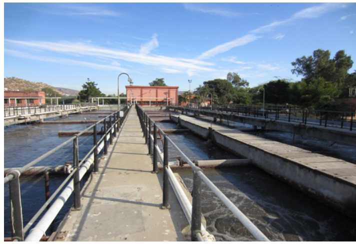
Figure 10.2 Conventional ASP to treat wastewater from the City of Jaipur (≈ 27 MLD).
