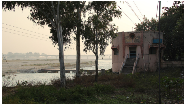
Figure 16.3 Example of a large diameter caisson well adjacent to Ganga River (Photo: HTWD, 2011).
