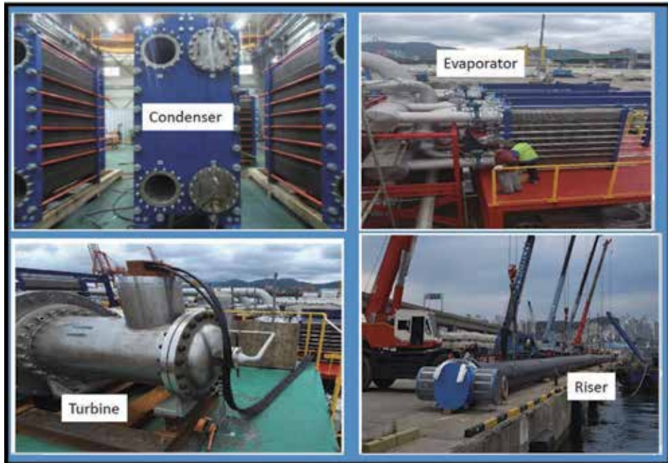
Figure 18. Key components of 1 MW OTEC plant of K-OTEC1000, which was loaded onto a barge ship for experimental tests, offshore from Busan, South Korea.
