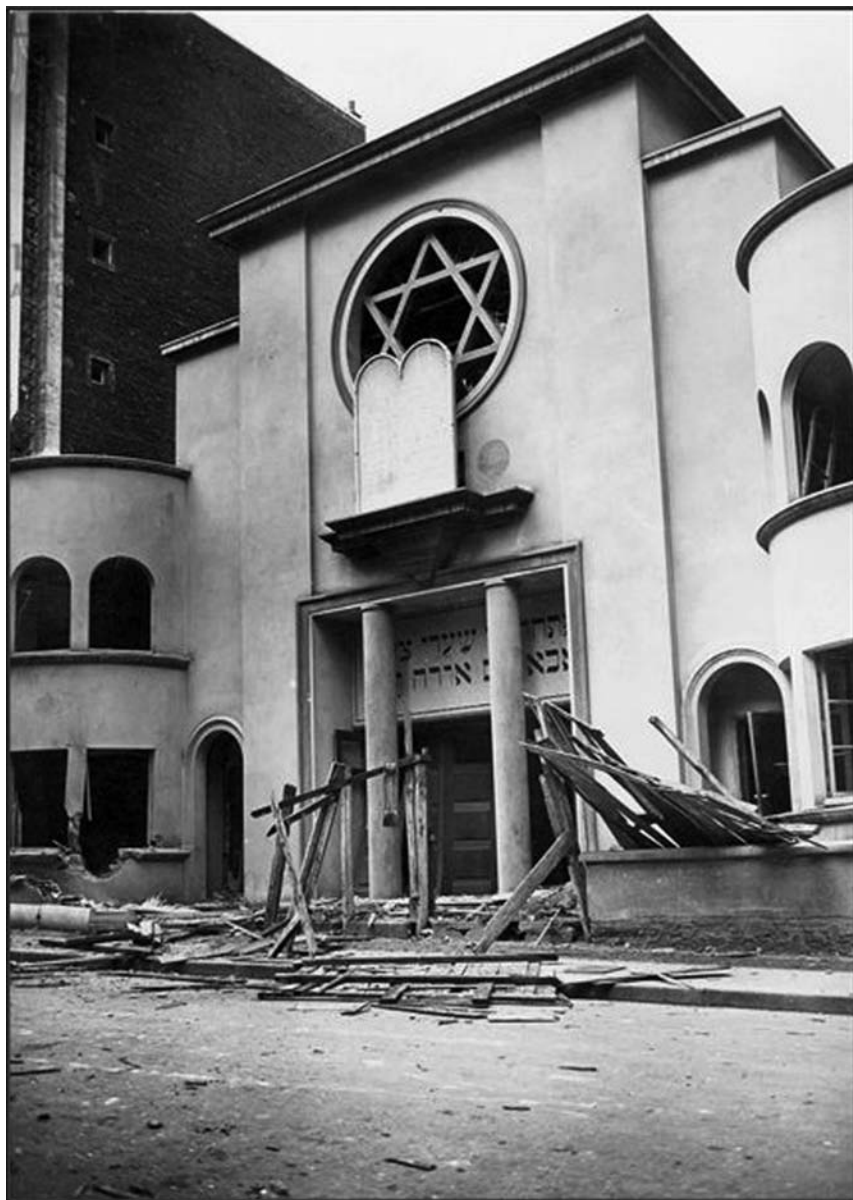
Figure 7: The demolished entrance of the synagogue on rue Sainte-Isaure
