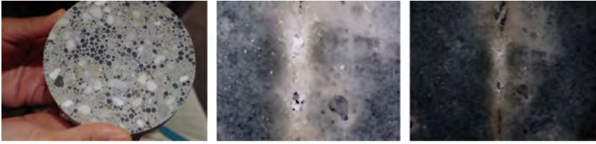
Fig. 5. Left: The bacteria and its food source, calcium lactate, are packed into tiny capsules that dissolve when water enters the concrete cracks. Once released, the bacteria consume the calcium lactate, creating limestone, filling in the gaps. Centre: bio-concrete healing process. Right: Bio-concrete healed (Greg Beach 2018)
