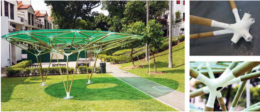
Fig. 6. Installed bamboo gazebo “Sombra Verde” and node close-ups
