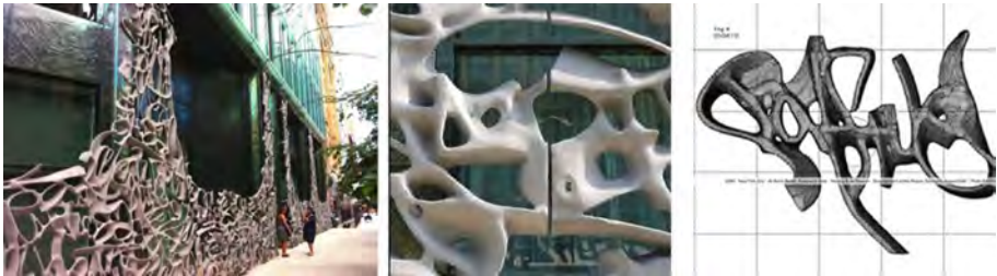
Fig. 16. Sculptural Gate at 40 Bond Street in New York ([Aluminum components] n.d. [image online] Available at: < https://www.exyd.com/40-bond.html > [Accessed 06 July 2018])
