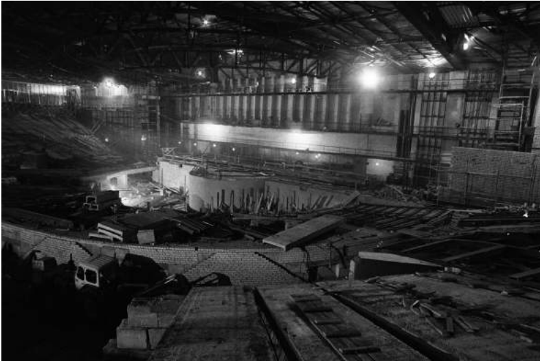
Fig. 4.3 Construction of Linnahall, 26 February 1980. Source: Valdur-Peeter Vahi, Rahvusarhiivi filmiarhiiv .
