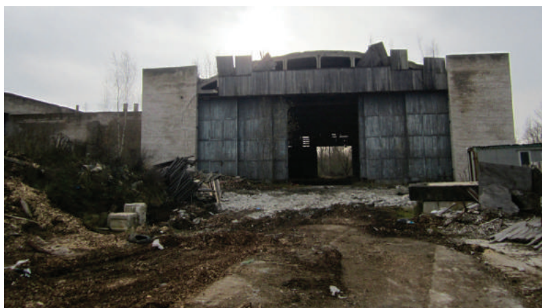
Fig. 7.1 Former hangar of the military airport. Source: Author, 2015.
