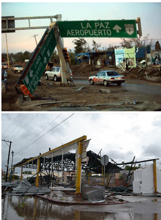
Fig. 14.1 Damage caused by Hurricane Odile in La Paz, Mexico (Source www.lacrónica.com , mmspress.com.mx )
