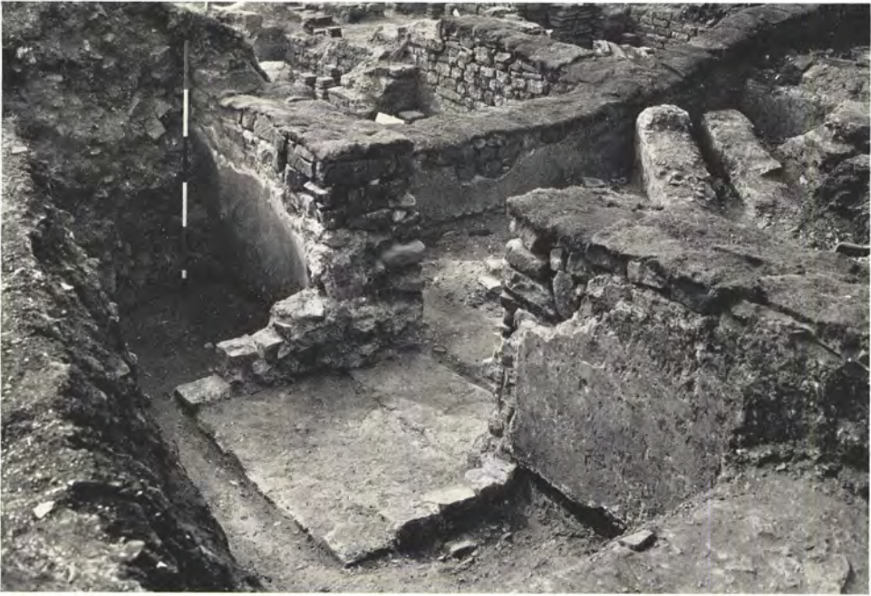
A. Exterior of room xxxvii in bath-building, showing small furnace and external rendering of painted cement. ( See pp. 54-5 )
