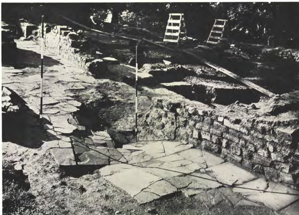
A. North-east ambulatory of temple, showing subsidence of secondary paving over swallow-hole. ( See p. 29 )
