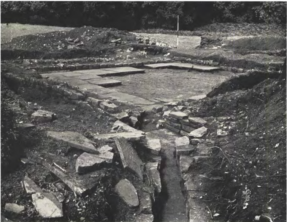
B. Tank and conduit. ( See p. 54 )
