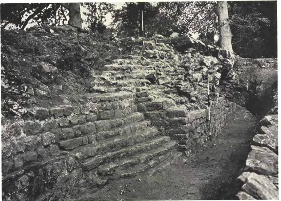
b. Precinct wall at south-east corner of 'guest-house'
