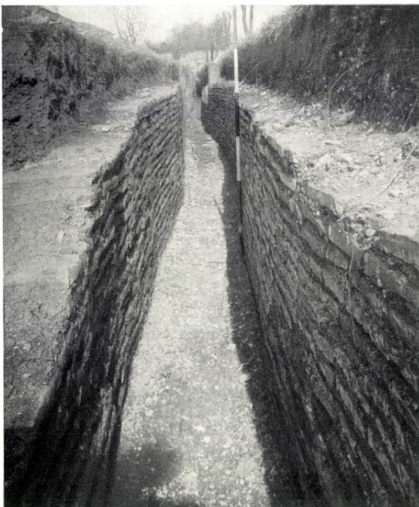
C. The same drain, looking north. [39], p. 88.
