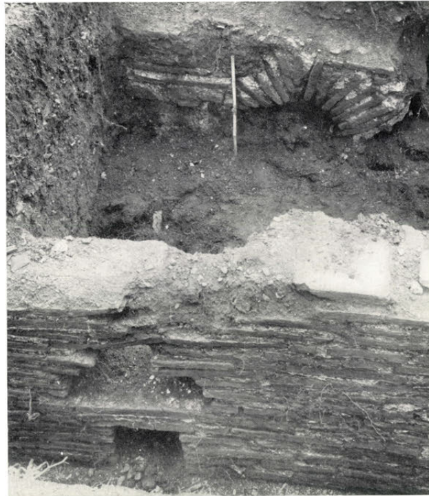
B. Openings in west wall of drain and arch in house-wall opposite near the NE. gate. [150], p. 88.
