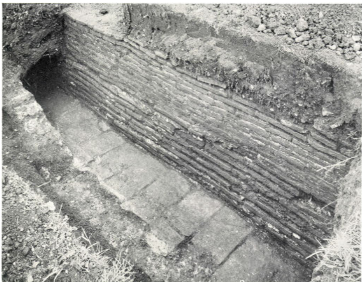
A. Drain, near NE. Gate, showing construction. [39], pp. 88, 89.
