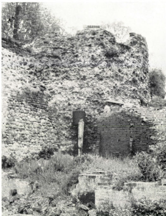
D. Bastion 1 from south. p. 45.
