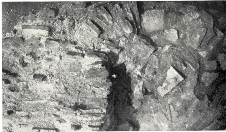
B. Fallen window-head at the NE. Gate. p. 39.
