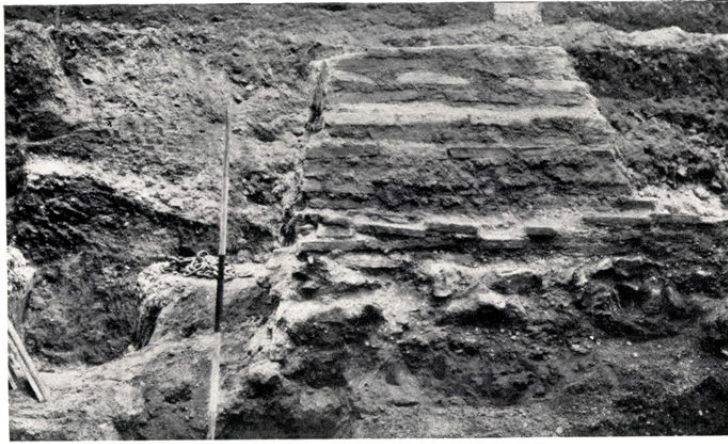
A. Pier of brickwork on stone foundation, found at St. Martin's House, 1950. [174], p. 98.
