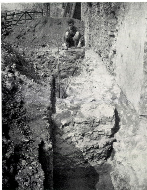
C. Excavation of foundations of Bastion 4. [147], p. 50.
