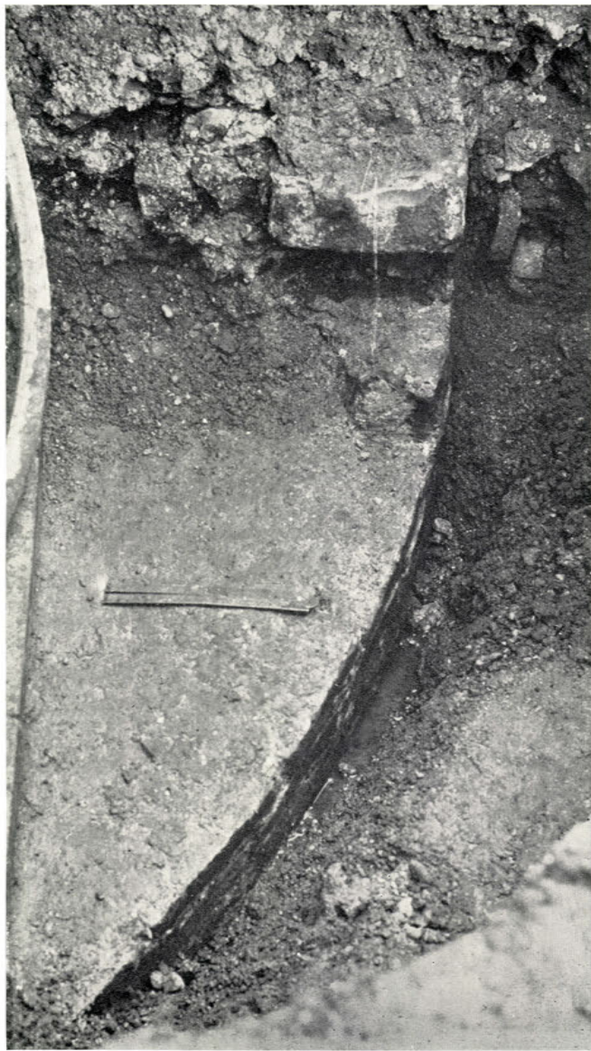
A. East side of North Gate, looking south. p. 32.
