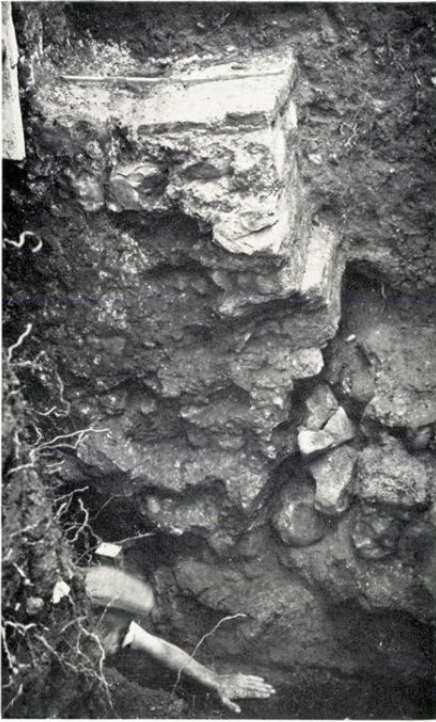
A. Broken foundations of Roman town wall. [104], p. 53.
