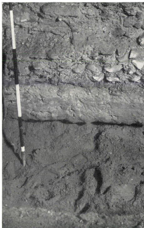
C. Foundation of central dividing wall between vaults. [34], p. 166.
