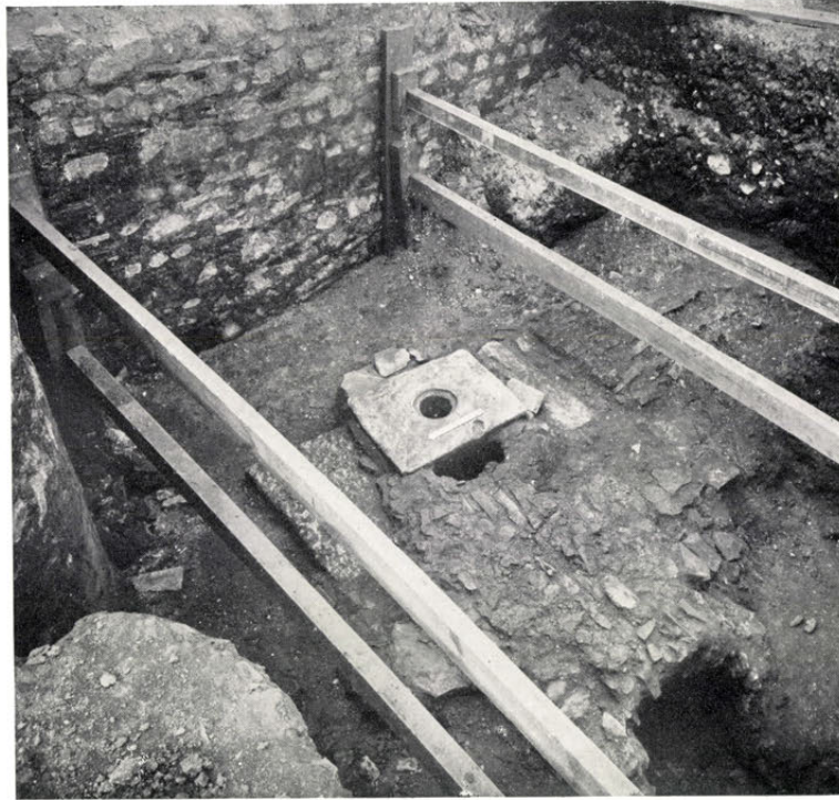
A. Roman drain and man-hole cover, south of Castle. [148], p. 175.
