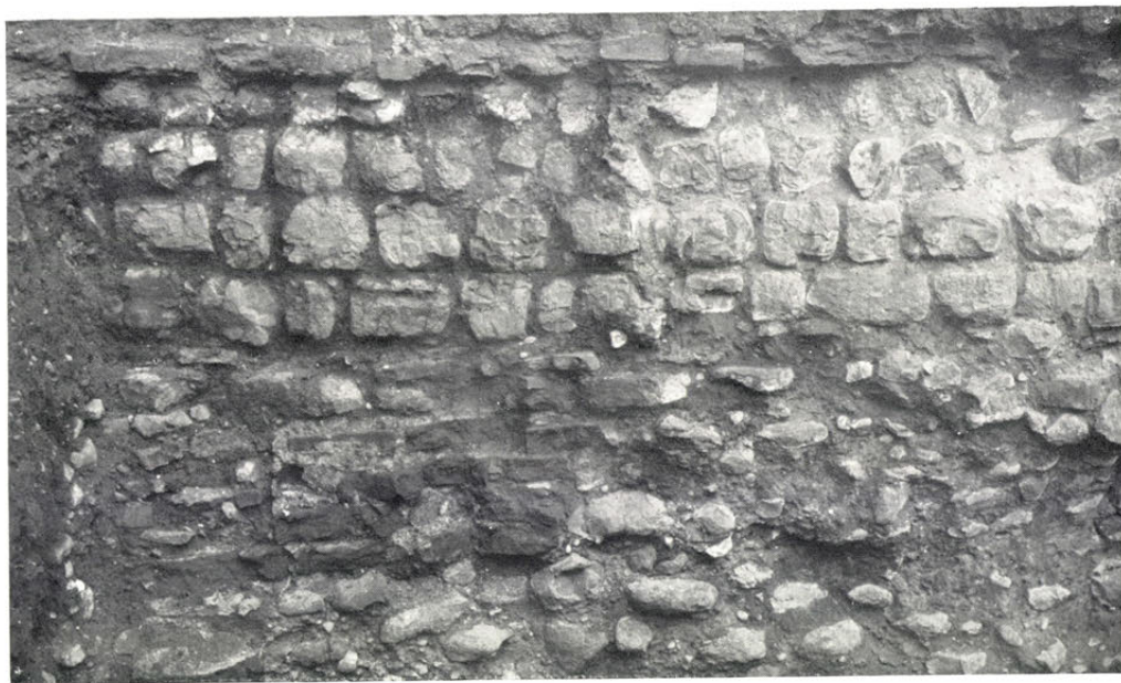
A. West face of cross-wall in Keep, showing tiling in the Roman work beneath. [34], p. 167.
