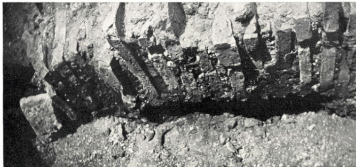
C. Fallen window-head at the NE. Gate. p. 39.
