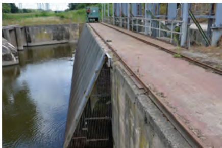
Figure 7. Existing industrial bridge with a cleaning machine.
