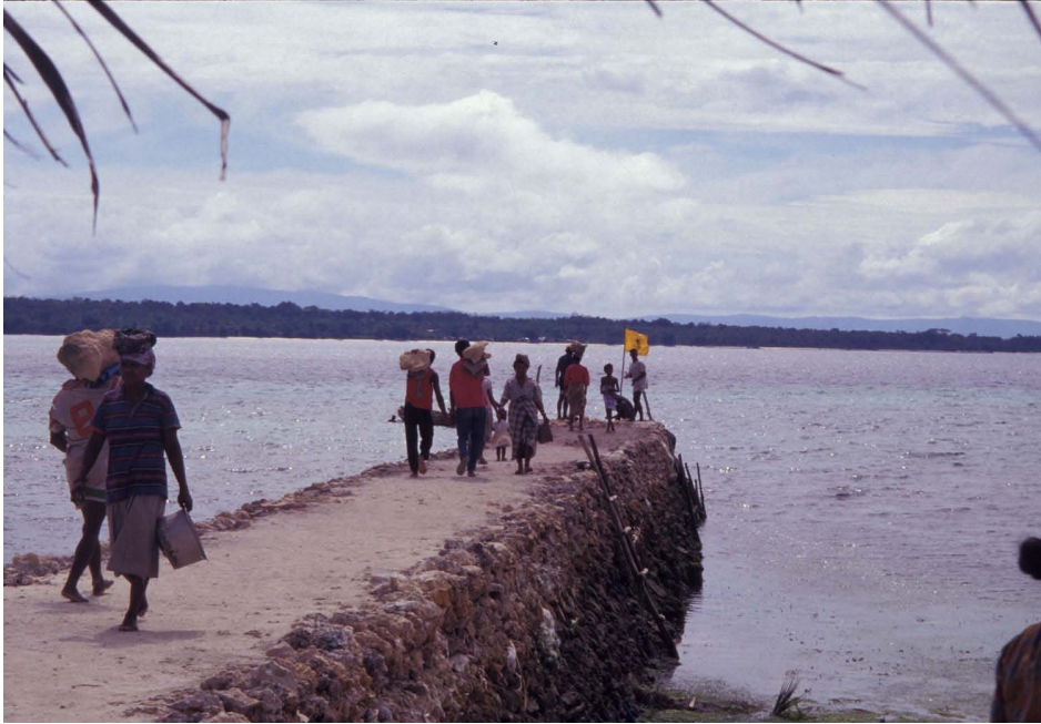
Plate 3-2: The under construction stone dock in Ohoislam (1996).
