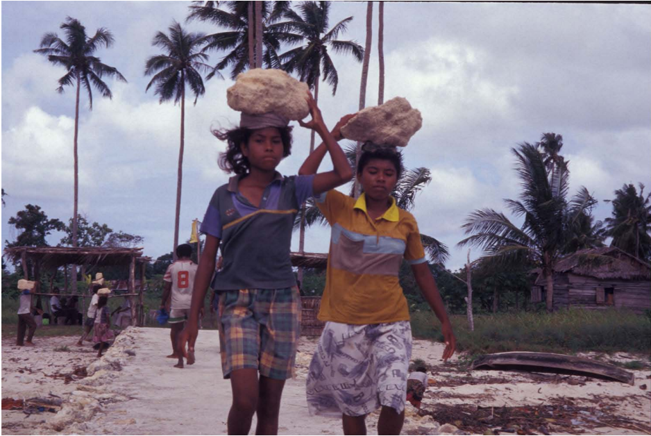
Plate 6-1: Two young girls help with the construction of the stone dock.
