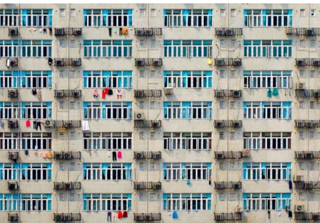
Haphazard and chaotic construction of slum-like apartment buildings Photo: Mark Tuinier/Flickr
