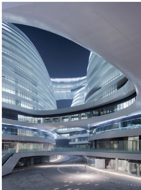
Galaxy Soho is a new office and retail and entertainment complex on the East Second Ring Road in Beijing. It was designed by Zaha Hadid and Ma Yansong of MAD Architects. Xi Jinping has publicly revealed that he does not like the ‘weird architecture’ of China’s modernising cities
