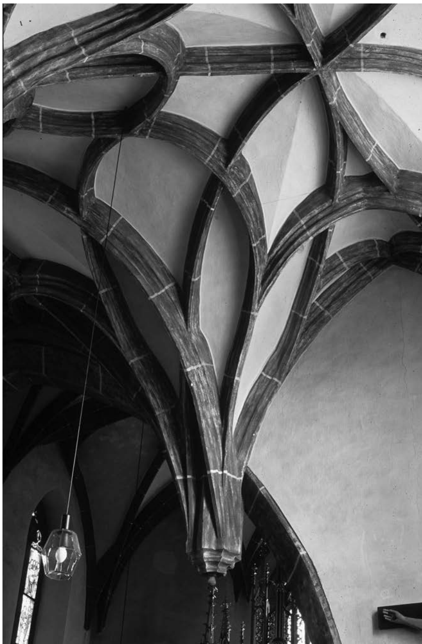
Figure 7. Parish Church, Weistrach, Ribs and Cone
