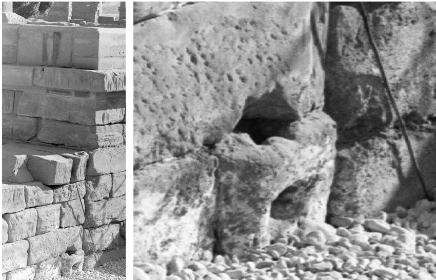
Figure 6 (left). North quay wall at Karnak showing the steps and two mooring loops (after CHEVRIER, 1947, pl. 48); Figure 7 (right). North-west corner of the western tribune with a mooring stone in the fifth course of the north wall (after 39685 ©CFEETK).
