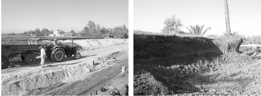
Figure 3. Wadi material is being used to level former Nile channels (left), whereas the banks of the former channels are being bulldozed (right) and the excavated Nile silts are being used as topsoil in the infilled channels. Pictures are taken 2 km south of Dayr al Barshā.
