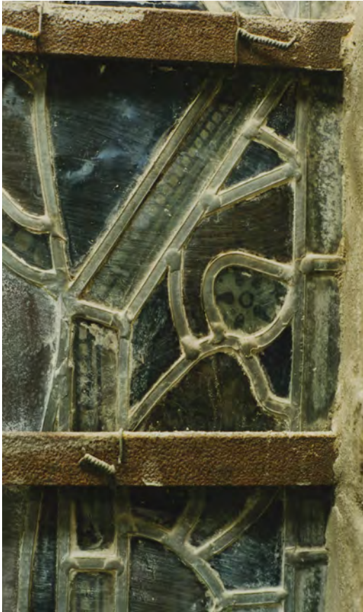
Figure 3. Detail of the exterior of the Bardi di Vernio window in Santa Croce. The smudges all over the window are the result of the first general cleaning of the window by the Polloni studio. The piece of glass at the left of the photograph, just above the metal tie-rod, is pitted from age and pollution. The newest piece of glass is the small triangular piece just below the tie-rod at the center-right of the photograph. Taken by the author from the restorers' scaffolding in 1997.
