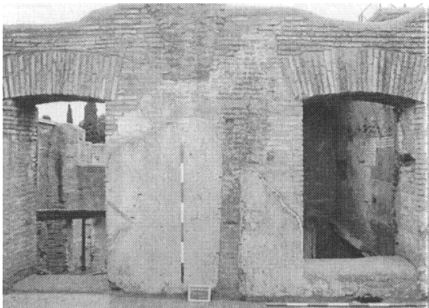
Figure 5.7 Marks of curtain wall in Rm 129.
