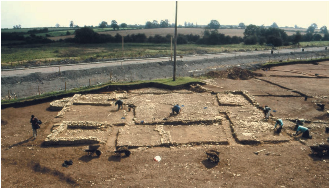
Plate 12: Tenement E, following removal of demolition rubble from the buildings and central yard
