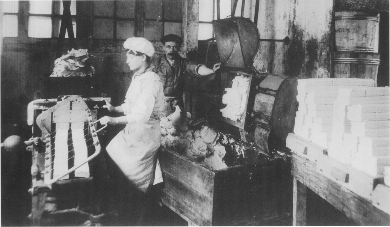
Figure 10.12 In 1914, there was a sudden influx of women into the margarine industry. This influx was related to introduction of a machine which looked like a large egg-slicer. The machine, shown here, cuts slabs of margarine into pieces of the same size. The invention made packing margarine much simpler. The photograph was taken in the Jurgens factory in Oss in 1914.
