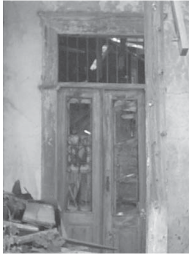
Fig. 4. Metal-clad Door Examples.
