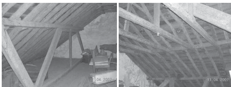
Fig. 2. General view of the structure.
