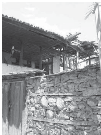
Fig. 3. The use of “hatil” – an example from Kula.
