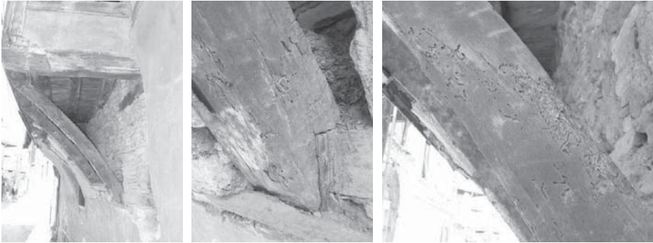
Fig. 6. The holes caused by insects – Example from Kula.
