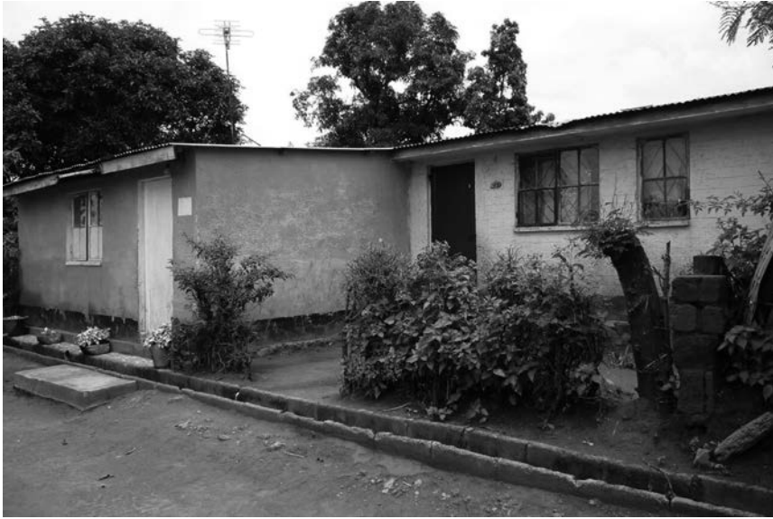
Figure 3.13: Transformation of an OCA house with an extra room added to the front, situation anno 2010.
