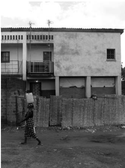
Figure 3.12: Enclosures in various materials in front of two-story houses with commercial shops on the ground floor, situation anno 2006.
