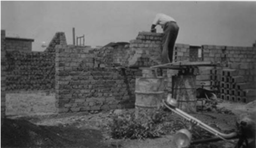
Figure 3.3: Building with the Système Grévisse in Lubumbashi.
