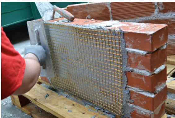
Fig. 2 Application of a PBO-FRCM strengthening to a masonry substrate
