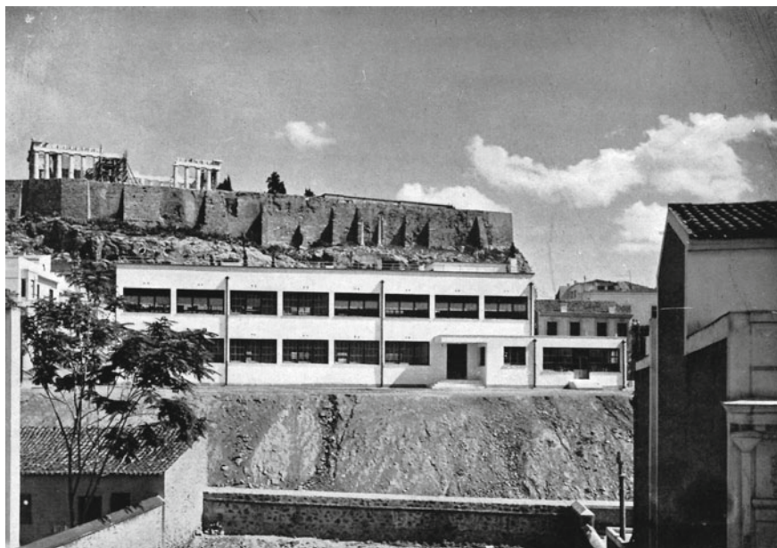
Fig. 3 Photo of school on Kalisperi Street, with the Acropolis in the background. Photo by P.M.Bardi (1933) from Quadrante n.5
