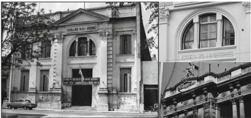
Fig. 10 Architectural elements composing the Morra's façade: tympanum, thermal window, pilasters in giant order, cornice
