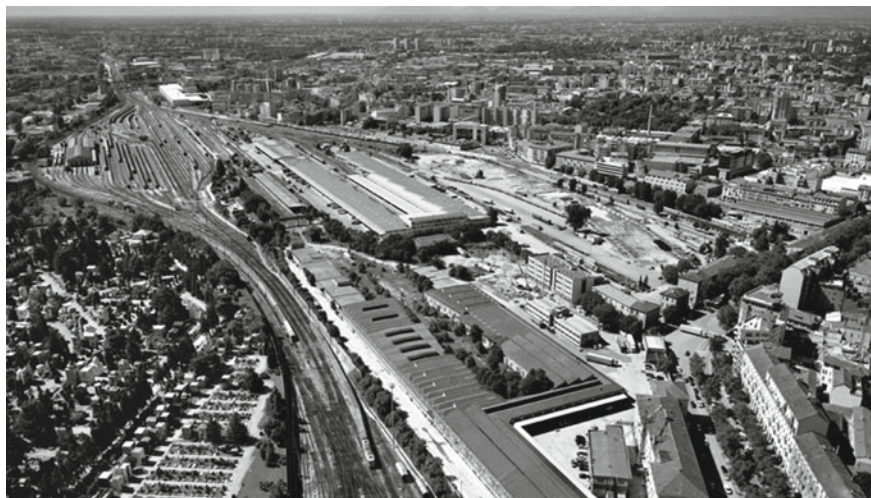
Fig. 1 Aerial view of the Farini marshalling yard, 1998. Photo S. Topuntoli
