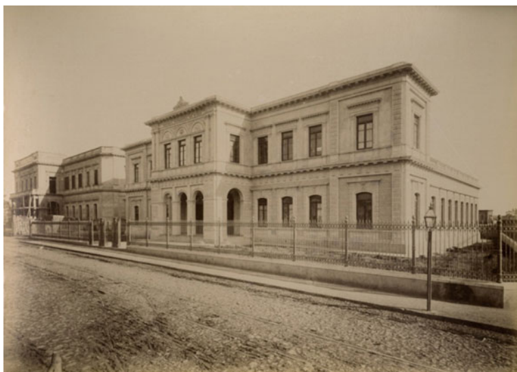
Fig. 1 Escuela Elemental de Niñas during their construction, photo S. Boote, 1889
