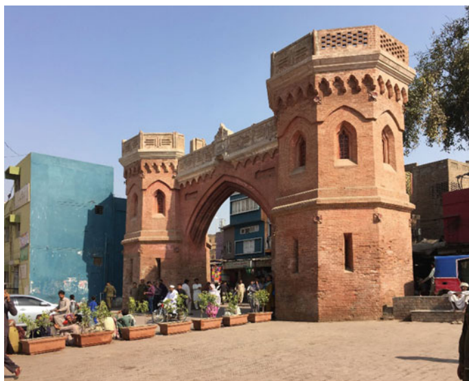
Fig. 3 Multan. Haram Gate after conservation work
