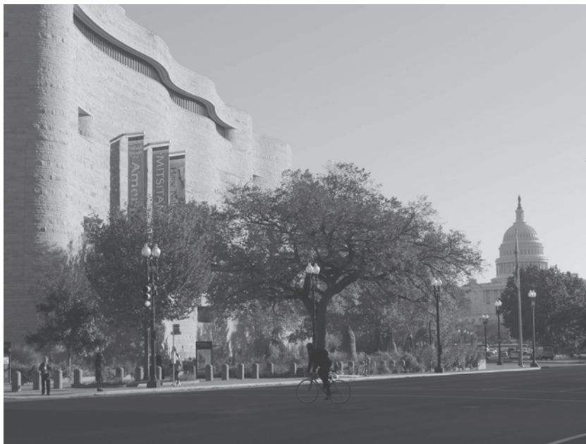
Figure 5.3. National Museum of the American Indian, Smithsonian Institution, Washington, DC, Exterior. Photograph by John Coe Robbins.
