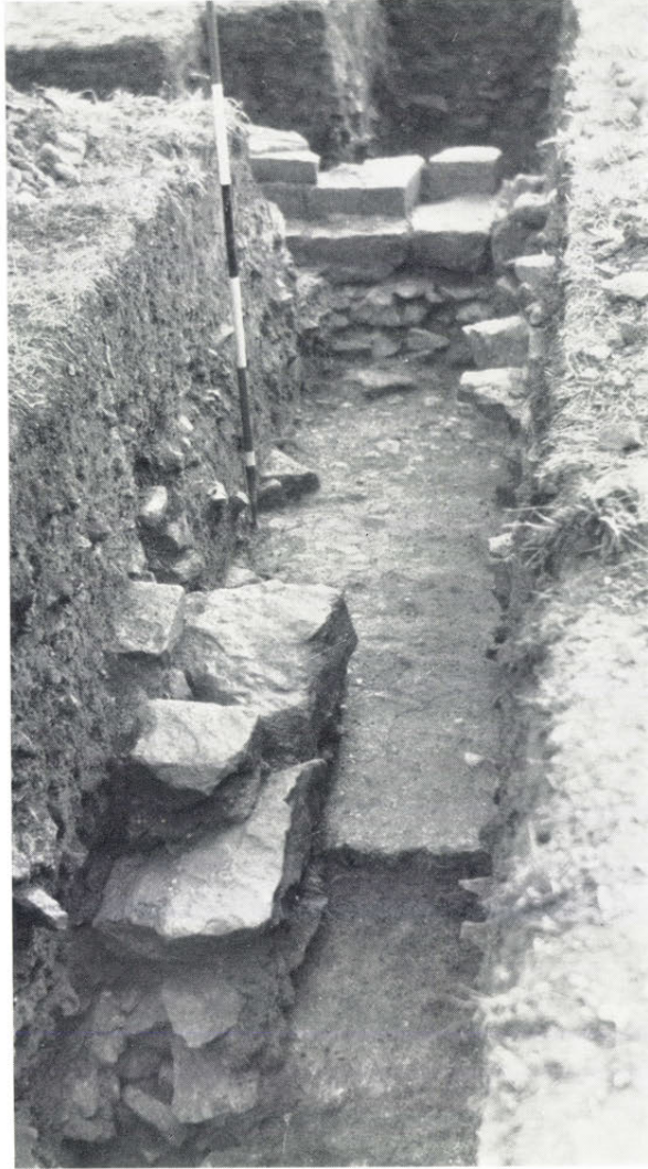
Gate-jambs and projecting imposts of the North Gate in Period VII
