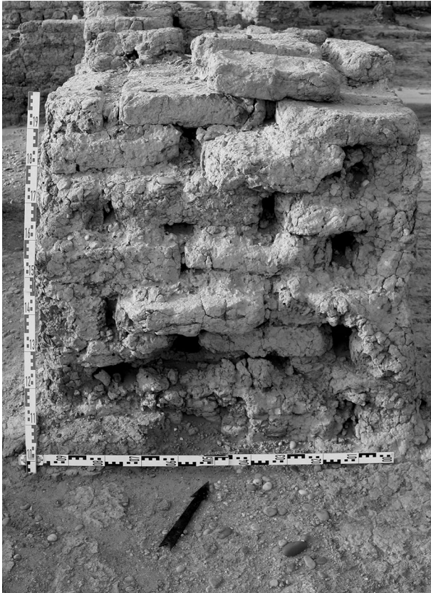
Pl. 13.1. Bricklaying technique – vertical section through a 1.06 m thick wall in SAF2
