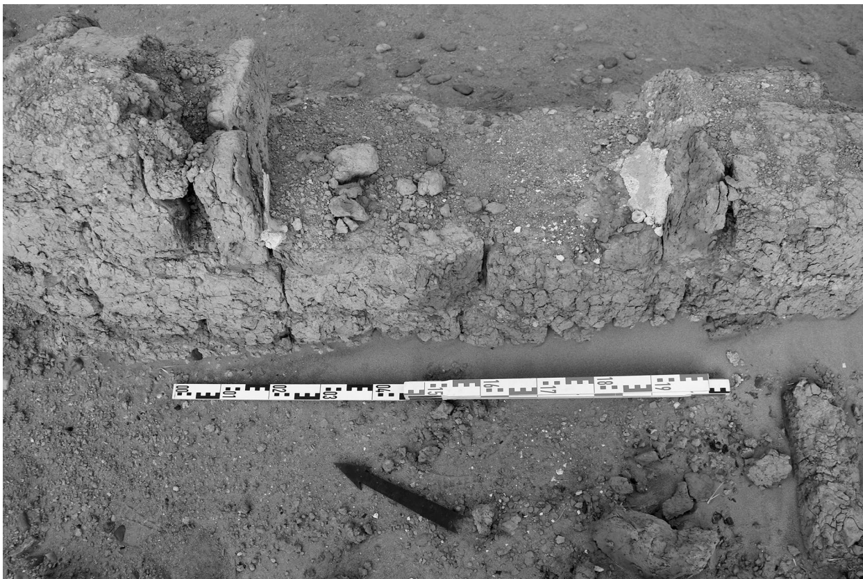
Pl. 40.1. Window in Room H3/2, view from the west
