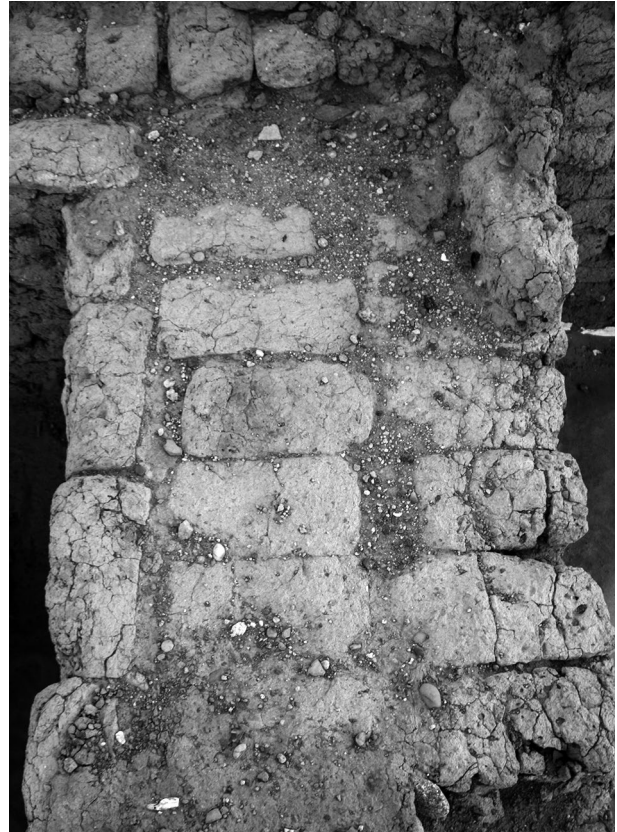
Pl. 13.2. Bricklaying technique – horizontal section through a 0.90 m thick wall in M14
