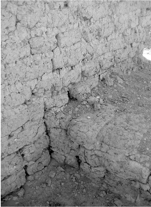
Pl. 45.1. Horizontal construction joint in Room SAF2/5
