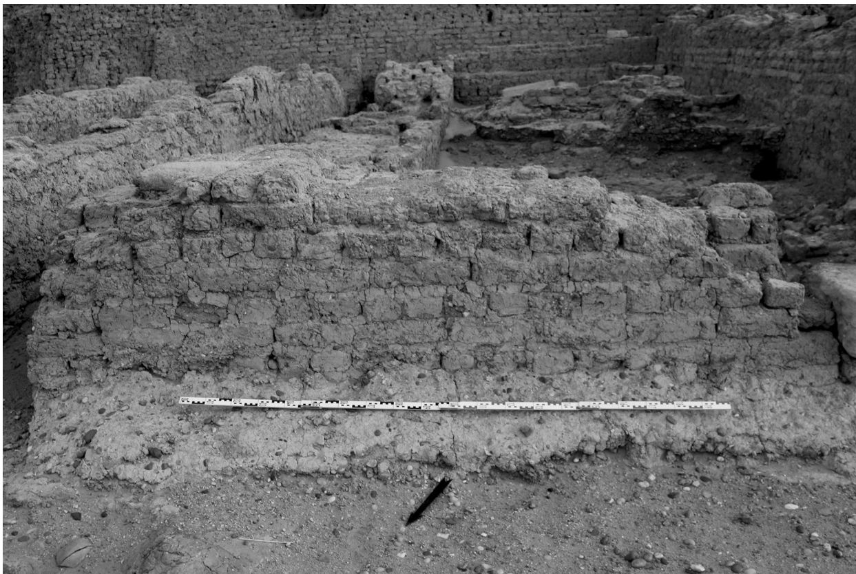
Pl. 14.1. View of the northern wall of the storage room M2 with a steadying method of the wall
