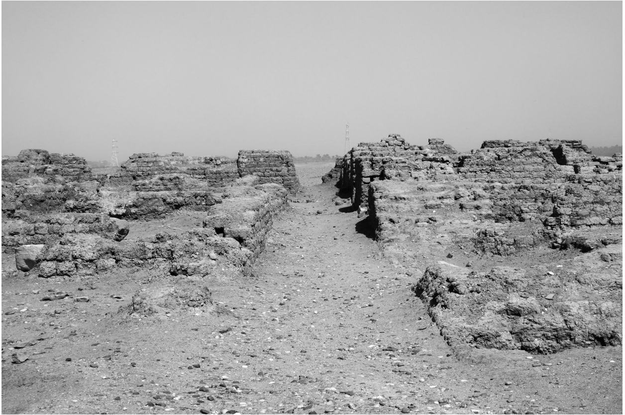
Pl. 21.1. Rue NS1, view from the south
