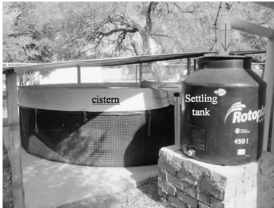
Figure 6.2 Typical above-ground cistern/storage and settling/sedimentation tank.
