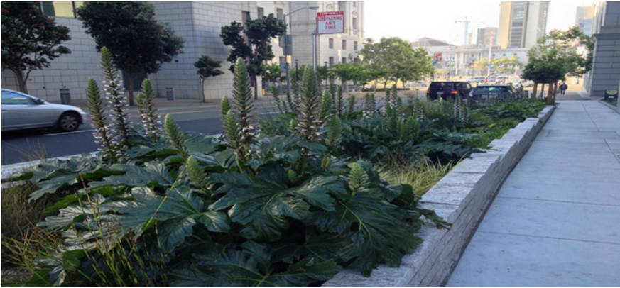
Figure 20.1 The ecological wastewater treatment and reuse system at SFPUC headquarters contains constructed wetlands that treat wastewater in the sidewalks surrounding the building.
