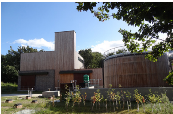
Figure 15.2 The OFWRP building and MBR activated sludge tank.
