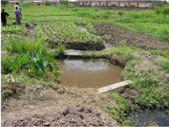
Figure 18.2 Simple sedimentation pond in an urban vegetable farm in Kumasi, Ghana (Photo: IWMI).
