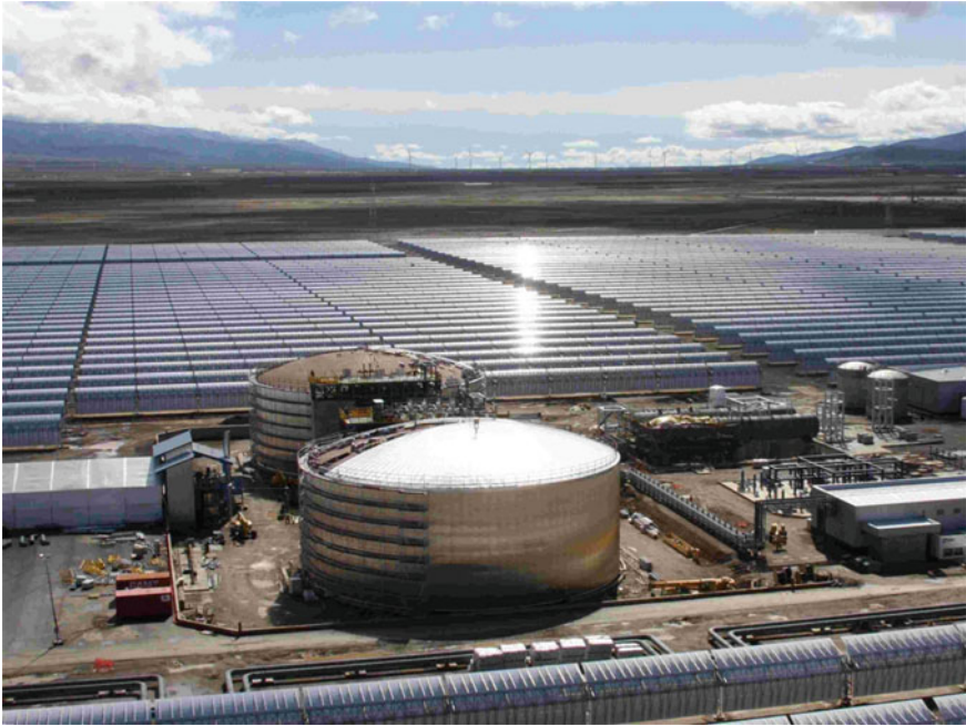
Fig. 3.16 A solar thermal power plant can deliver electricity on demand 24 h a day. Instead of expensive batteries for electricity storage, it stores thermal energy in tanks filled with liquid salt. One of the two storage tanks is filled with “cold” liquid salt at 290 °C. During the day, the salt is pumped through a solar powered heat exchanger and stored in the second, “hot” tank at 390 °C. During the night, the hot salt is pumped in the other direction to produce electricity on demand. The cooled salt is stored back in the first tank [65]
