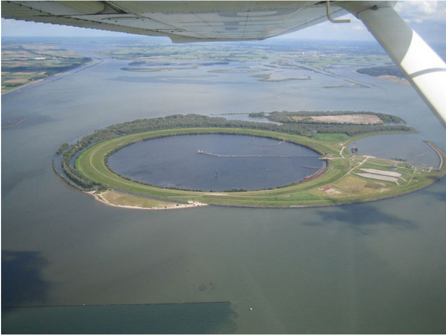
Fig. 3.15 An Artificial Energy Atoll can be used as base for off-shore wind power plants and as location for HVDC converter stations for undersea cables. The lagoon can be pumped out and used as pumped storage hydropower and as tidal power plant. The photo shows an example of an artificial atoll. This one is not used for energy but as depository to store polluted silt [63]
